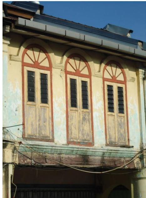
The trademark pre war shop houses with long wooden widows are dying (or rotting) out fast and literally falling apart, and being replaced by aluminium and glass ones.
